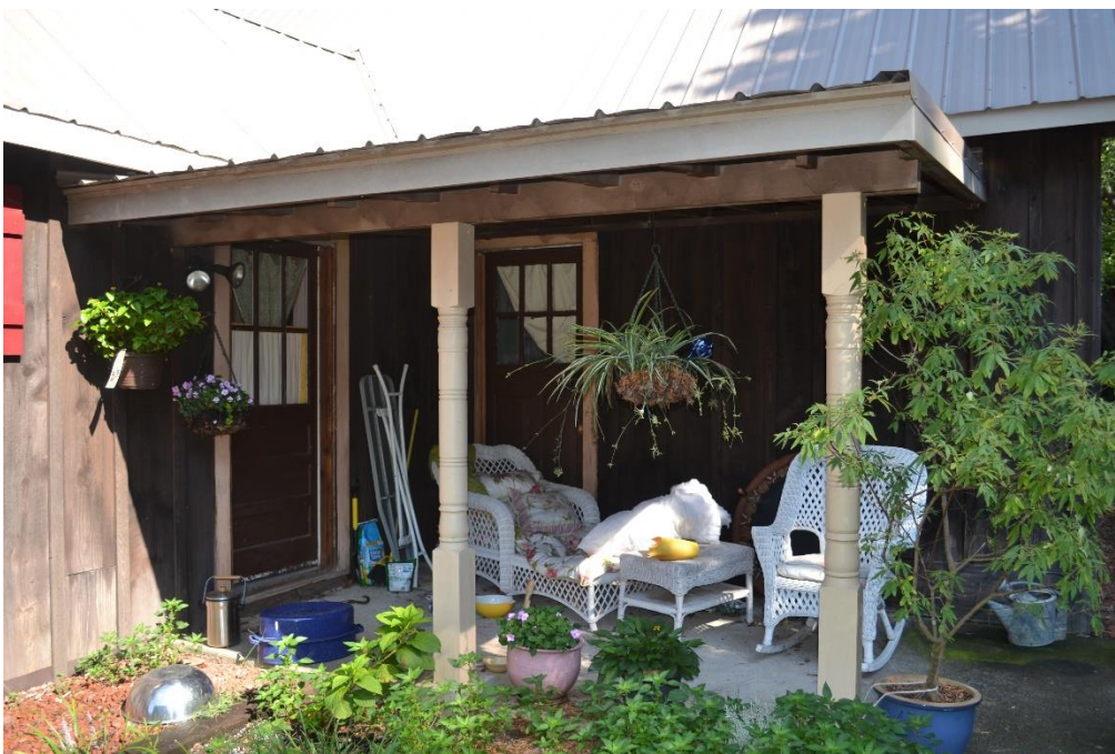
Mitchum-Hensley House, Front Porch, Looking North.
